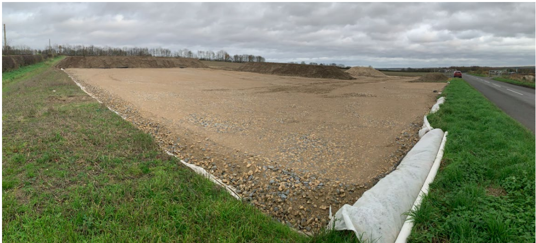
Photo 44: Example of a temporary construction compound
