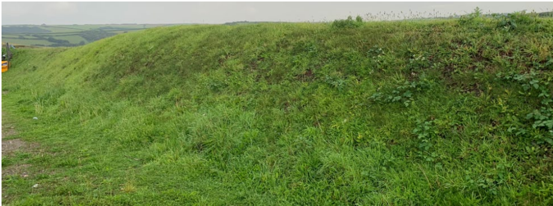
Photo 36: Grass-seeded Soil Storage
