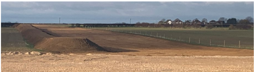
Photo 45: Example of a temporary bund (example shown for a water pipeline project)
