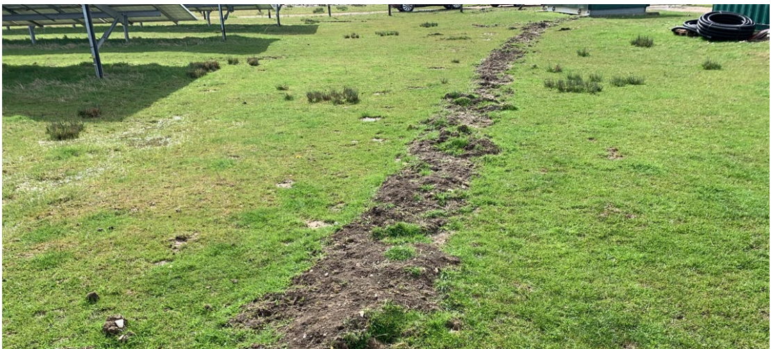
Photo 50: Trench During Wet Period
