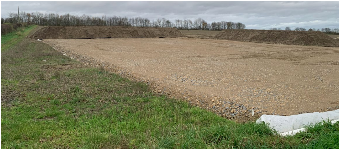
Photo 33: Newly-laid Construction Compound (Elsham-Lincoln Pipeline)
