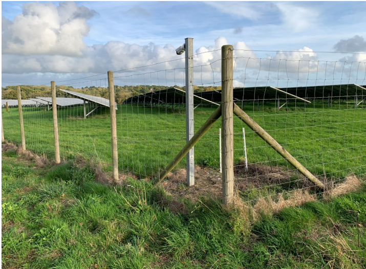
Photos 42 and 43: CCTV Poles and Fencing
